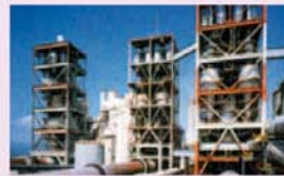
Raw materials for cement
