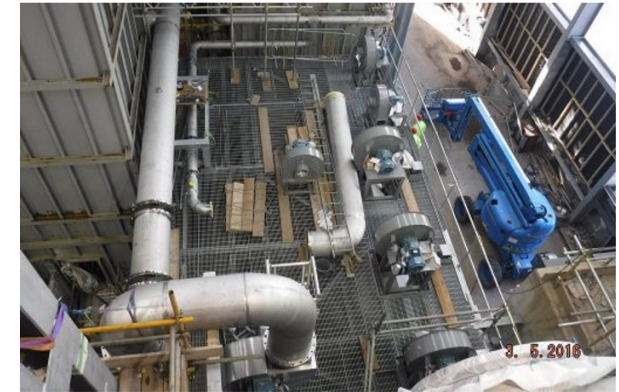
The gasification technology being installed at the Glasgow EfW build
