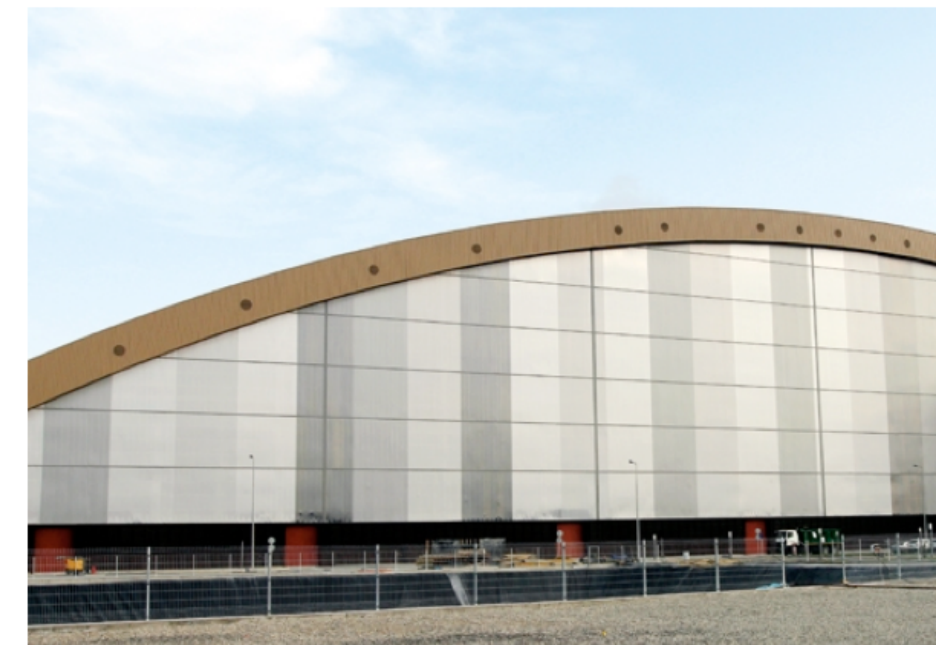
The Baku WTE plant (500,000 tons MSW/year)
