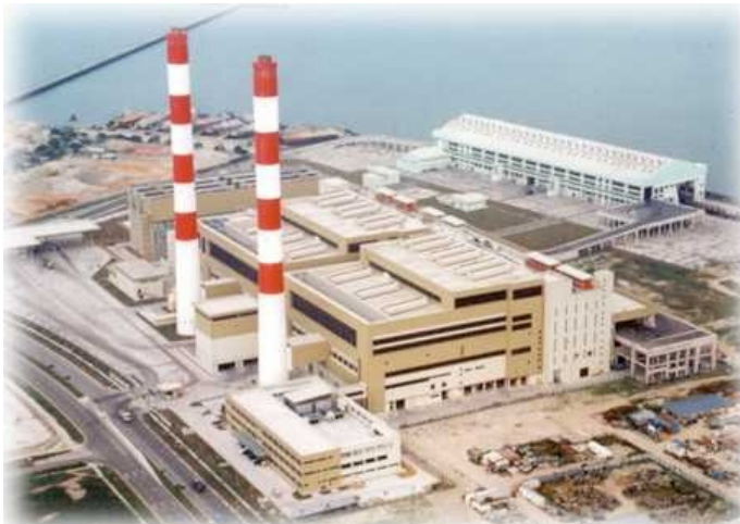
Tuas South Plant
