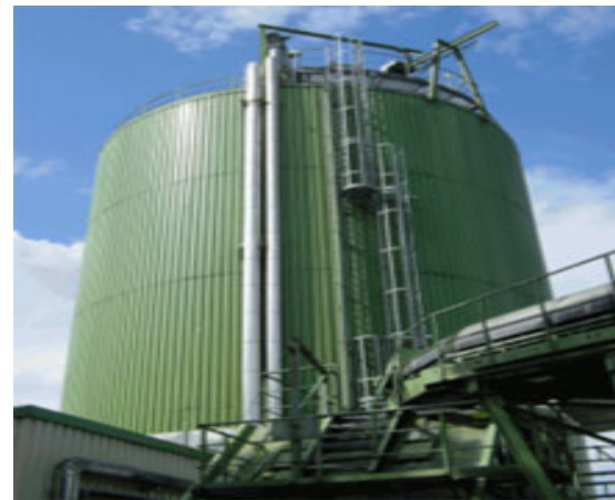
Food Waste Recycling Plant
