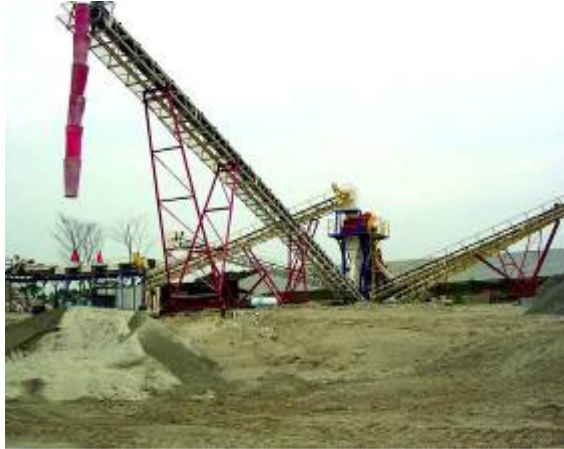
Construction waste recycling plant
