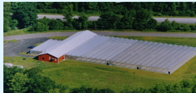
Burlington County Research and Demonstration Greenhouse
