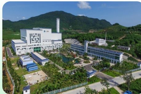
Boluo Waste-to-energy Project
