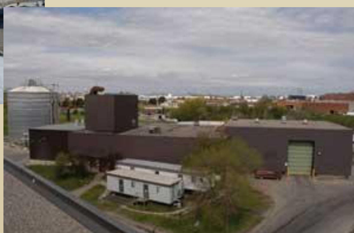
DOPF receiving and processing buildings
