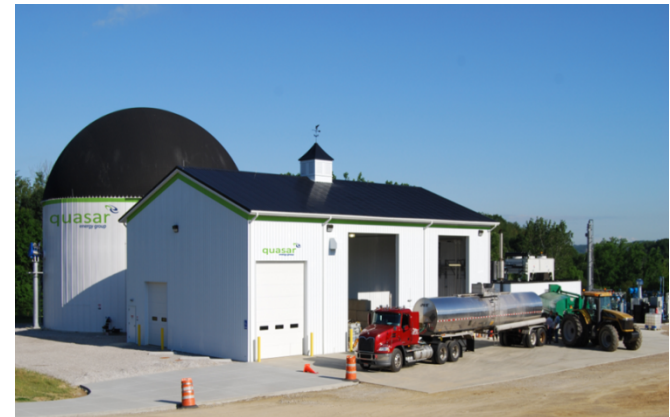
Wooster, OH- 20,000 TPY, Pumpable and high solids organic biomass
