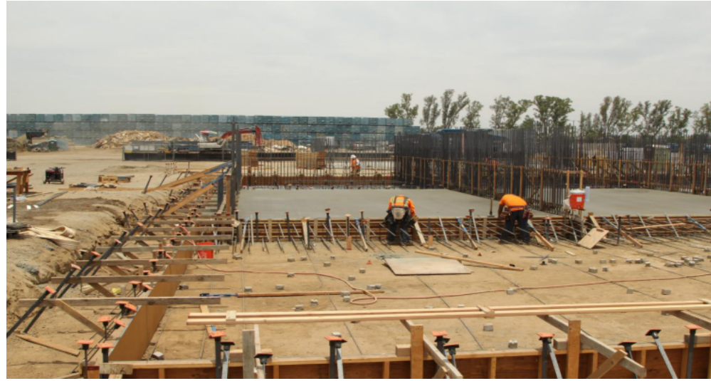
CR&R Eisemann – Perris, CA (under construction)
