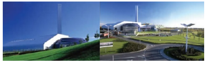
FIGURE 7. Two views of Brescia WTE facility in Italy.
