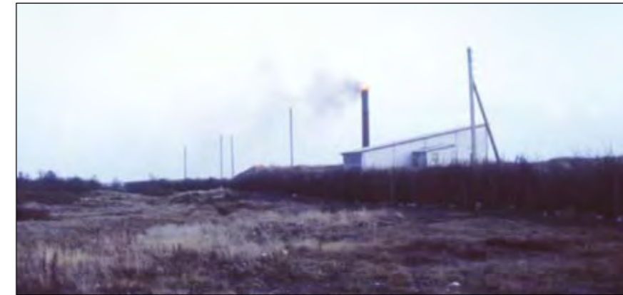
This photo taken around 1970 shows an incineration plant in Skagen (The Skaw) on the most northern tip of Jutland. The plant did not recover the energy produced and was therefore located in a remote area. As can be seen, the 'afterburning zone' was located on top of the stack. Plants of this type were targeted by Guideline no. 3/1986 issued by the Danish Environmental Protection Agency. However, the Municipality of Skagen prevented any intervention as in 1979 it replaced the plant shown by a new, still existing, district heating producing incineration plant supplied by B&S.
