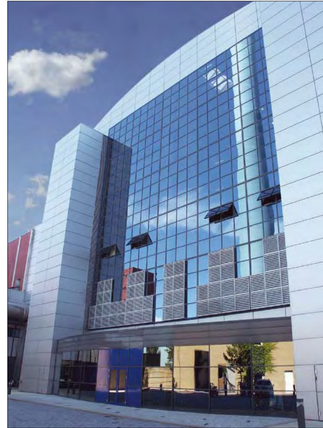
I/S KARA in the municipality of Roskilde: New combined heat and power plant commissioned in 1999. Consultant: Rambøll. Architect: Tage Niensens Tegnestue.
