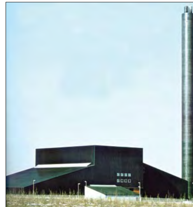
Aarhus Nord incineration plant, 1978. Architects: Friis & Moltke A/S. The plant was given its original name (Aarhus North) due to the plans also to build a plant in the south end of the municipality. But instead, a third unit extended Aarhus Nord in 1992, and a new unit 4 will be ready in 2005.
