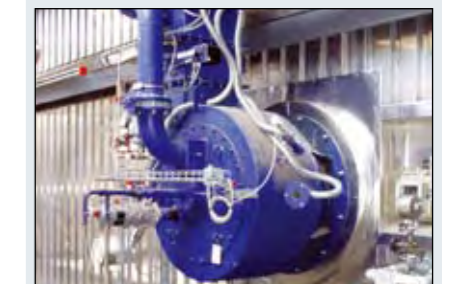
Start-up and auxiliary burner.
