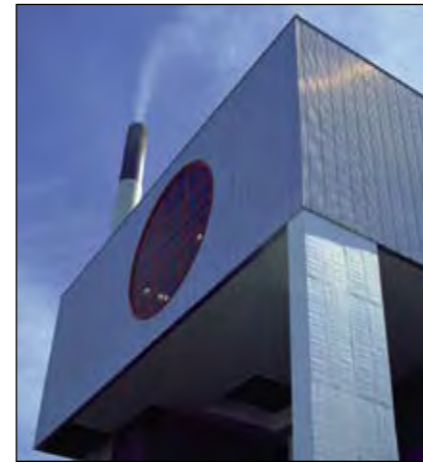
Amagerforbrænding. Architect: Jørgen Maglebye.
