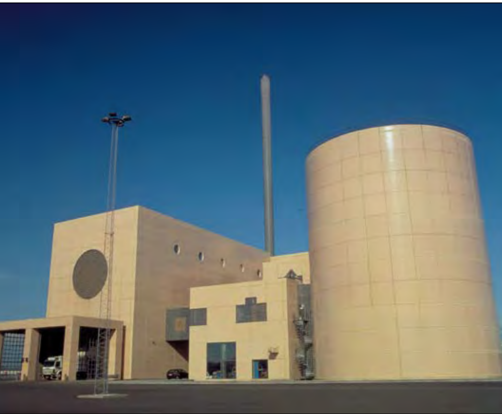
CHP plant in Horsens in Jutland, established in 1991. Architects: Boje Lundgaard and Lene Tranberg.
