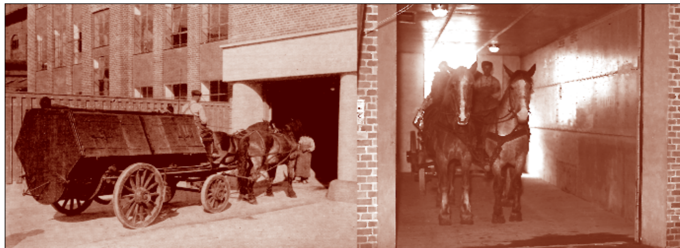
Horse-drawn wagons at Aarhus incineration plant. The wagons were taken up and down by lifts.
