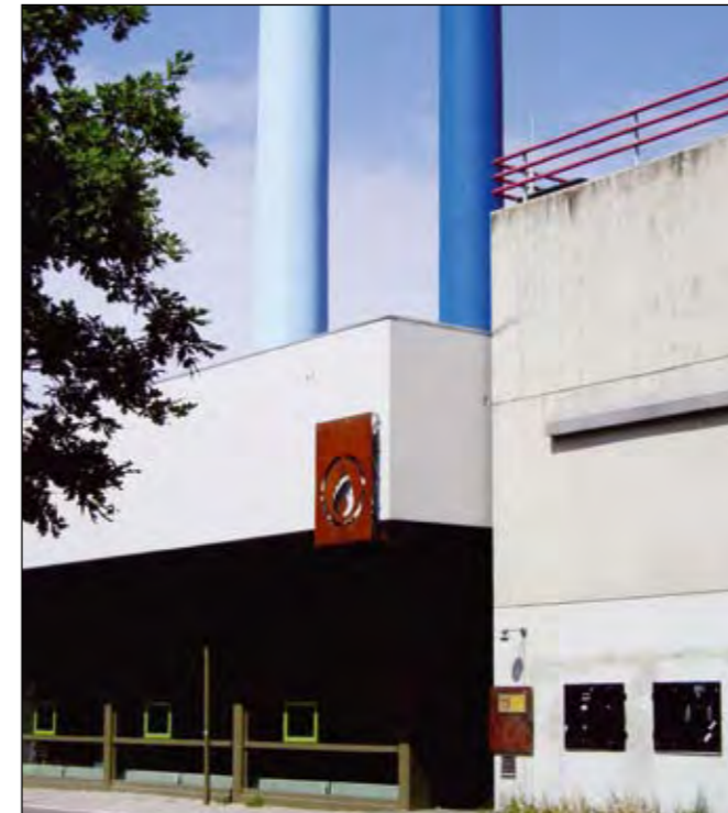
Albertslund district heating station. Architects: Friis & Moltke A/S. The building previously housed an incineration plant, too. This part of the building is now used as a regional music and culture centre called 'Forbrændingen' (The Incineration Plant).
