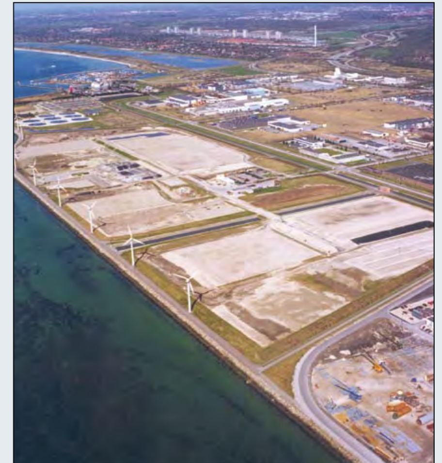
Sanitary landfill of AV Miljø, which is jointly owned and operated by Amagerforbrænding and Vestforbrænding.
