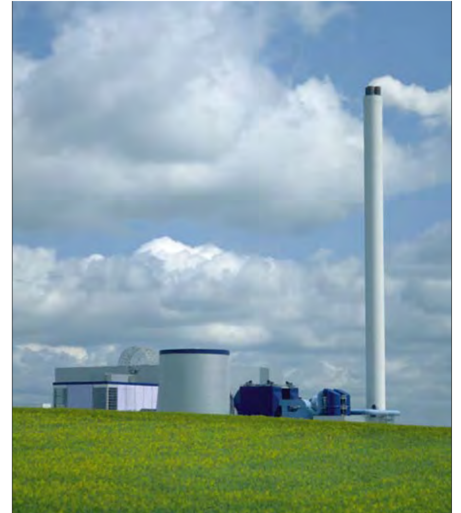
Måbjergværket in Holstebro in western Jutland. Architect: Torsten Riis Andersen. The plant does not only incinerate waste, but also straw. The steam produced is superheated in natural gas fired superheaters before it is applied for combined heat and power production.
