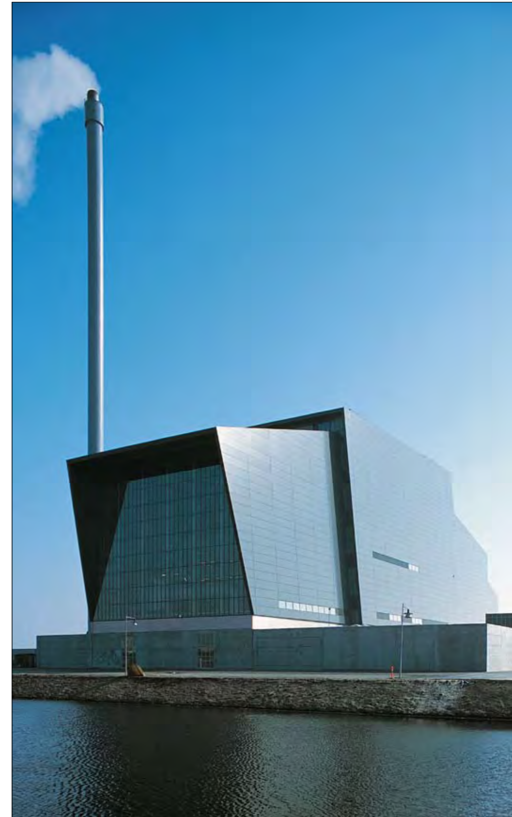
L90 - waste incineration plant in Esbjerg. Architects: Friis & Moltke.
