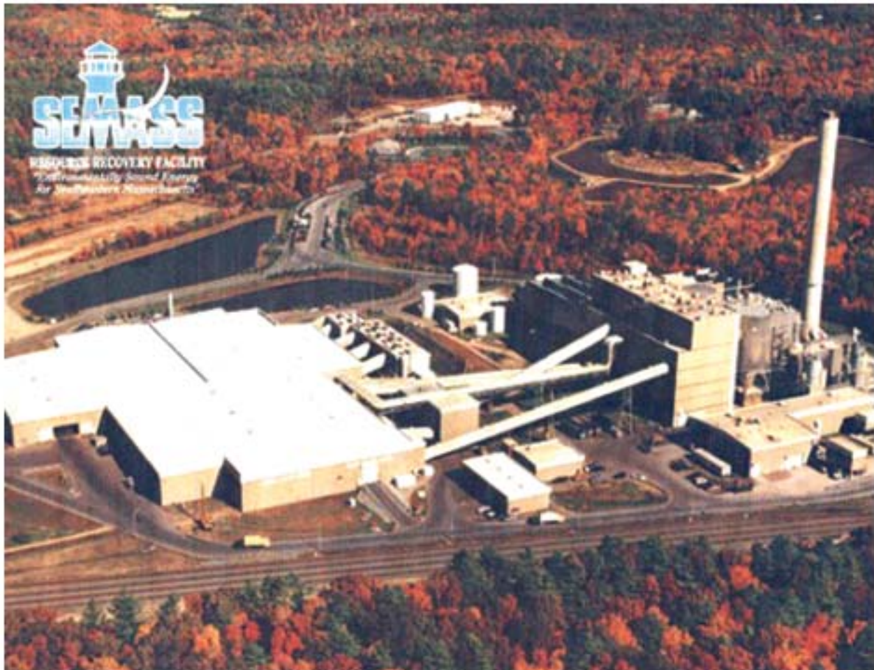
Figure B-5. SEMASS Resource Recovery Facility (Rochester, MA)
