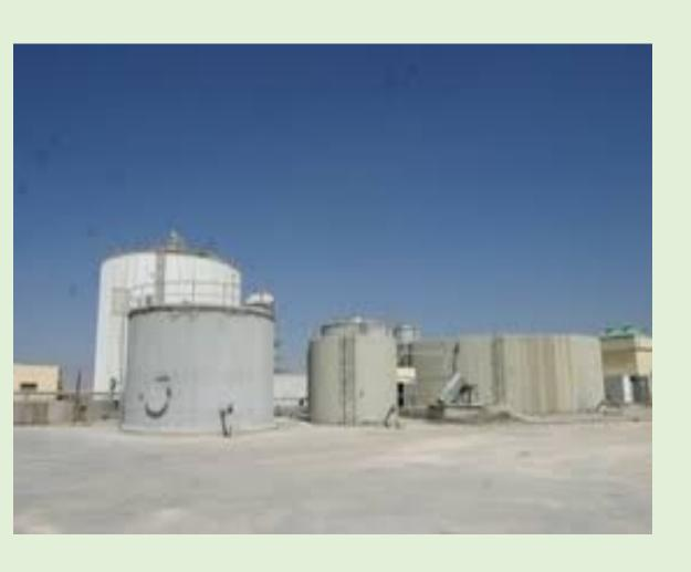
Electricity generation from waste digestion started taking place in Jordan in the year 2001. Anaerobic digestion demonstration plant with 1MW capacity was built nearby the closed landfill in Russaifah. The plant capacity has been increased in 2008 to about 4 MW..
