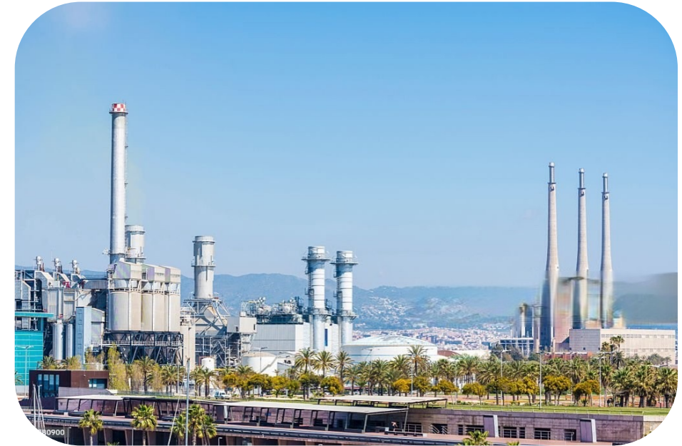
Incinerator plant in Barcelona
