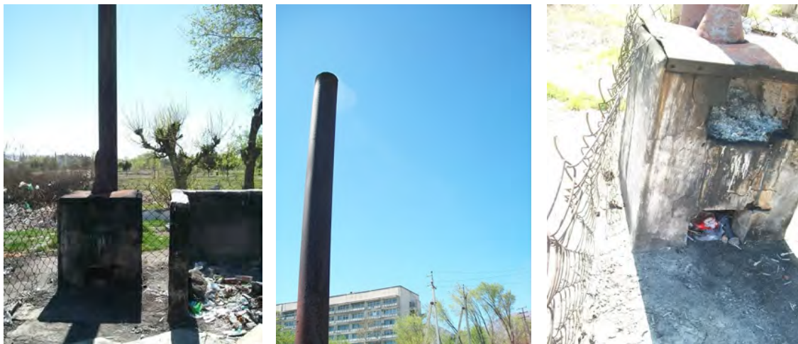
Figure 23: Oven for Burning Syringes at the Regional Hospital in Khujand
