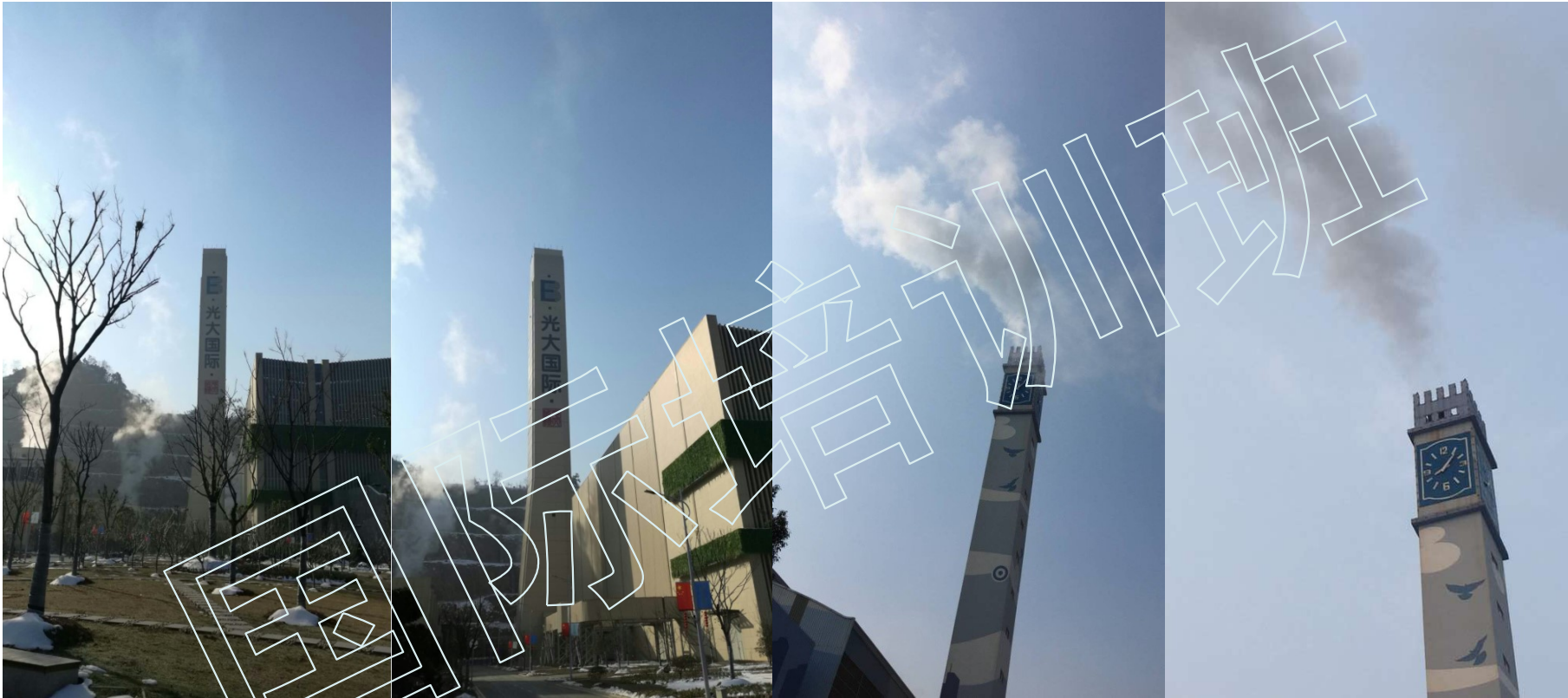
有脱白的项目与无脱白的对比 different projects with/without demisting
