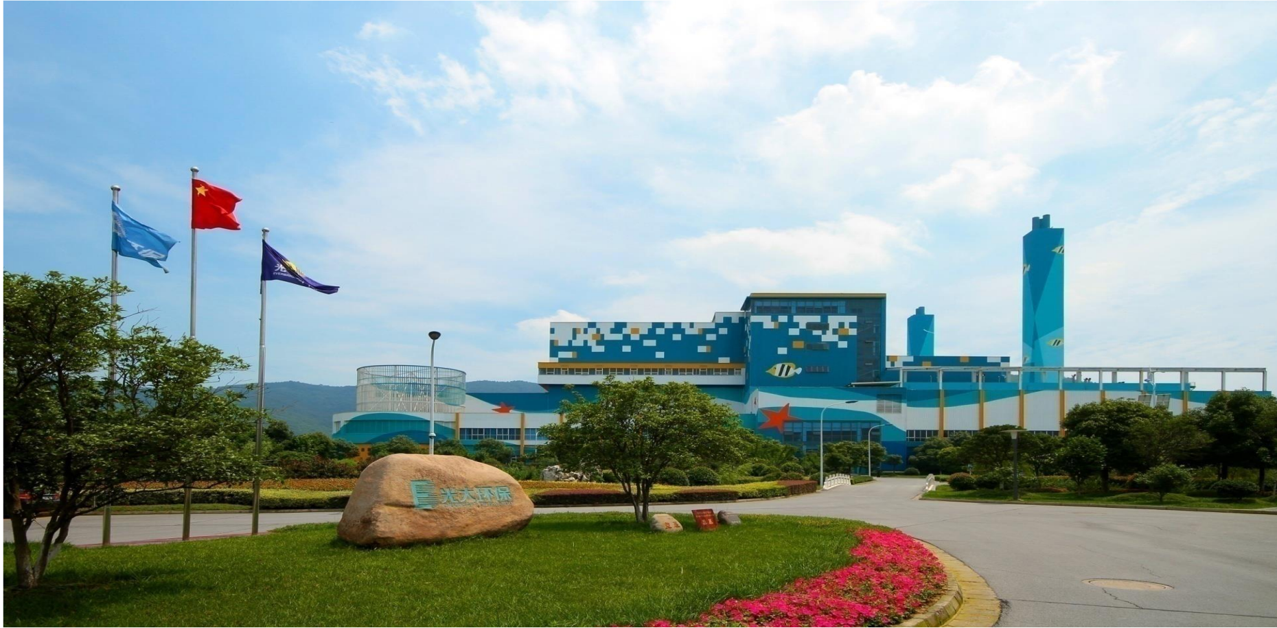
Suzhou municipal solid waste incineration power generation the third-stage project (3*500t/d)
