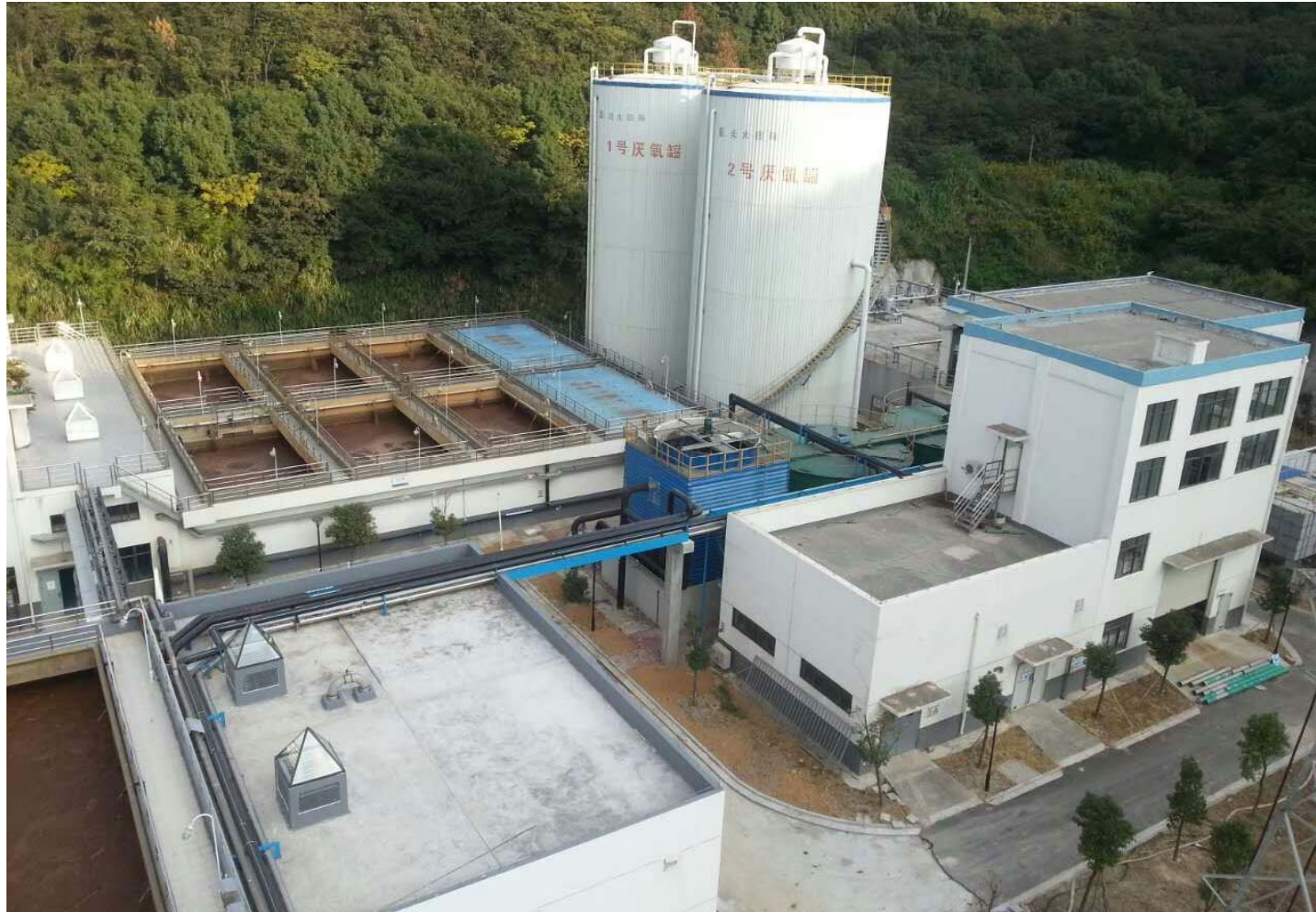
Leachate treatment in Ningbo waste-to-energy plant
