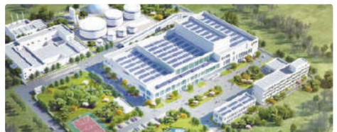
Shandong Ji'nan Kitchen Waste Resource Utilisation Project
