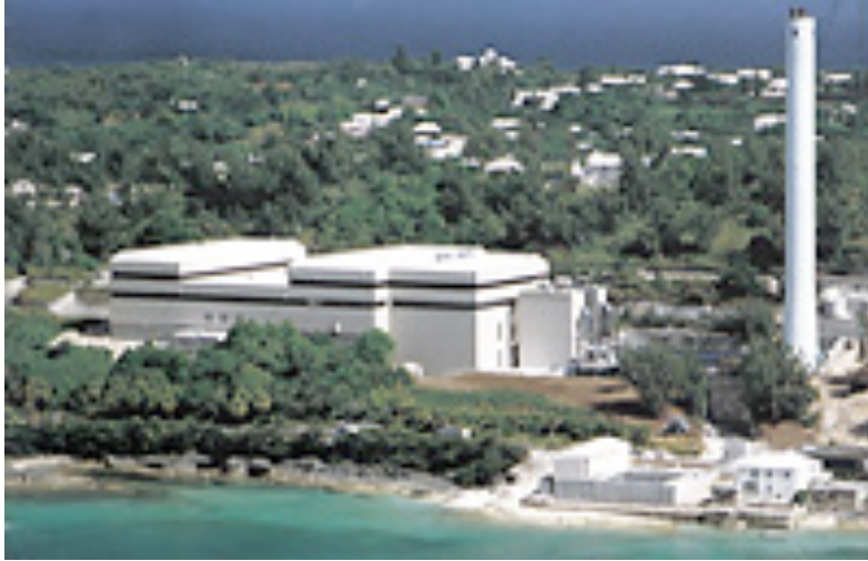
Figure 61 Tynes Bay waste treatment facility 85 (EEC)
