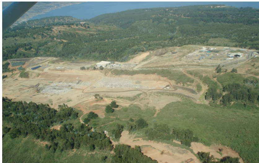
Figure 43 Aerial photo of the El Molle landfill (EEC)
