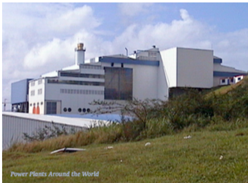
Figure 63 The Martinique WTE plant 92 (EEC)
