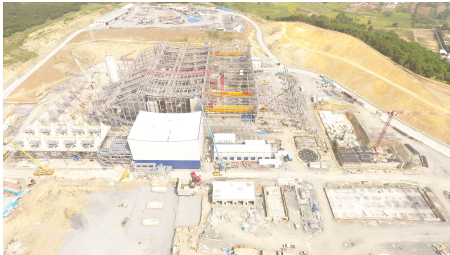
Figure 2. WtE plant in Istanbul, under construction [2]
