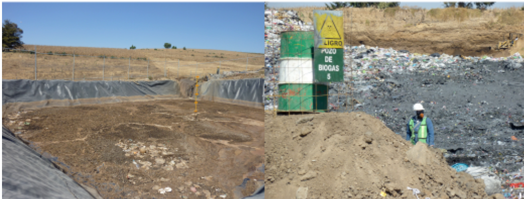
Figure 51: Leachate holding tank and LFG extraction well.
