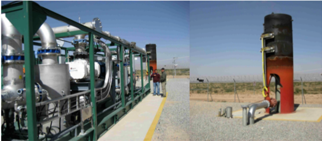
Figure 30: Ciudad Juarez sanitary landfill installations (M2M, 2009)
