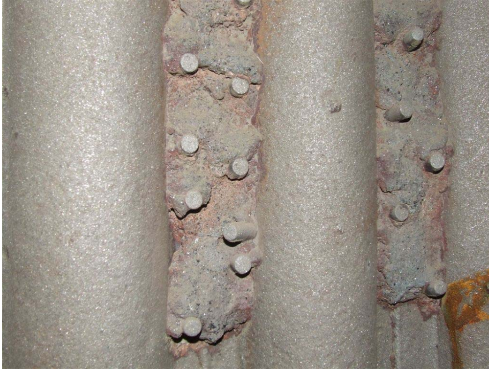
Figure 5. Studs and refractory in area to be cladded
