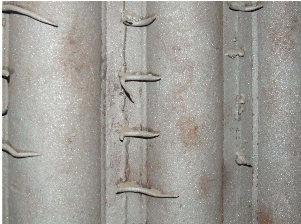
Figure 4. Refractory anchors in area to be cladded
