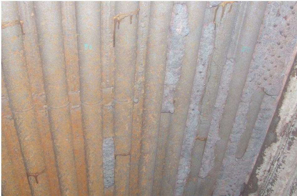
Figure 6. Large area with refractory obstruction in area to be cladded
