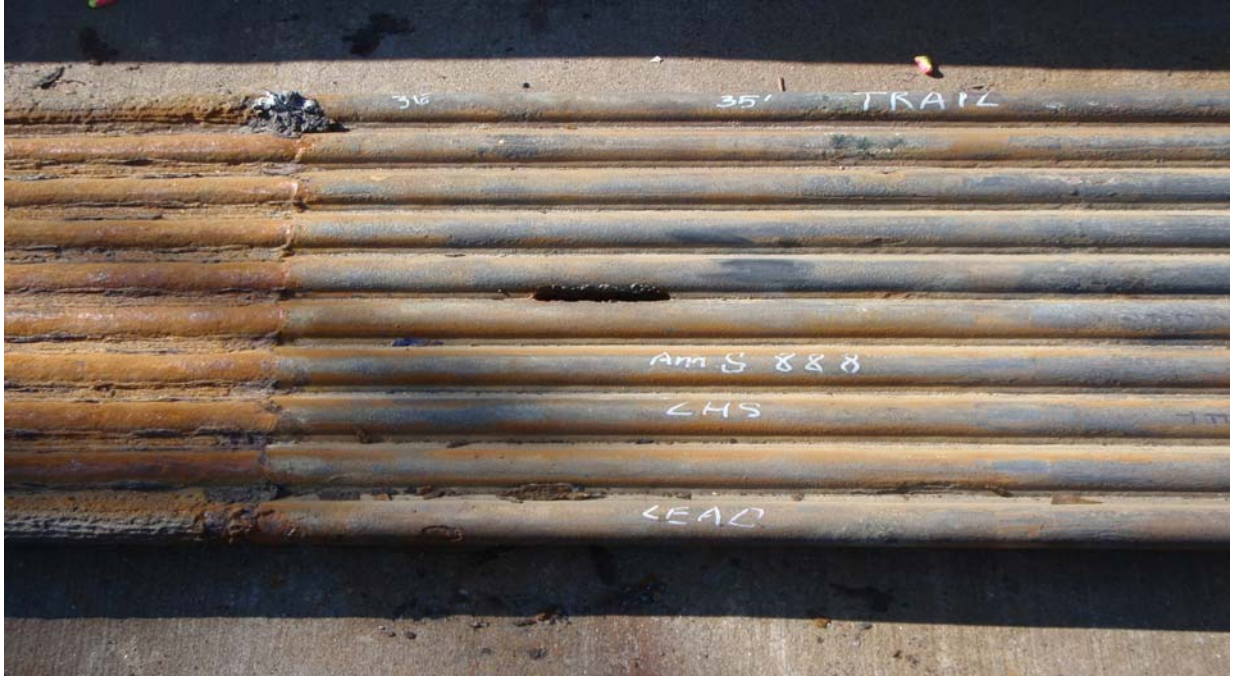
Figure 13. AmStar Panel 3-4 after 2 years of operation at 35' from Roof welded to non-trial panel with Inconel 625 weld overlay for the lead and trail tubes and 8 unprotected SA-213T22 tubes.
