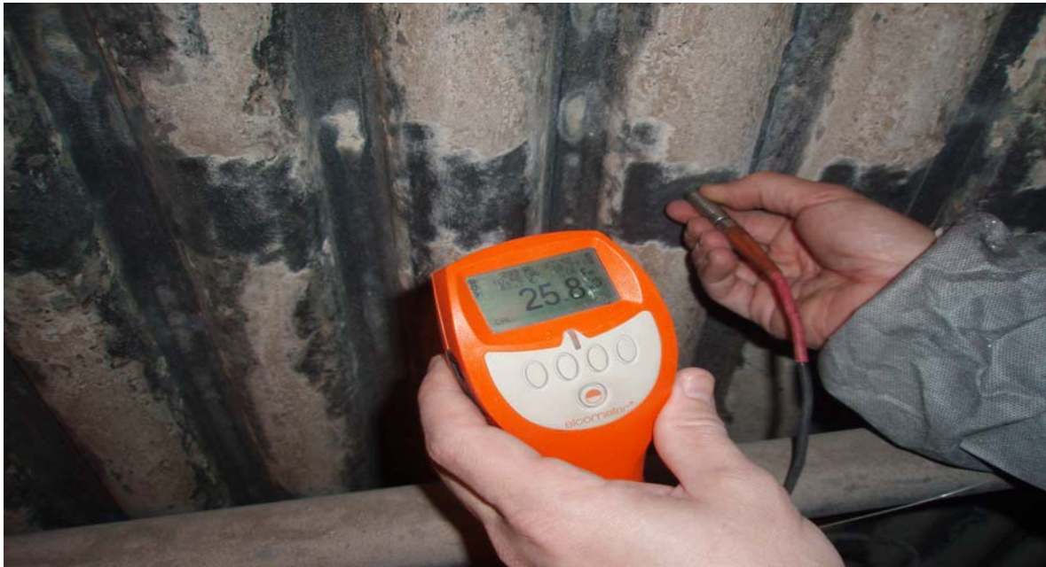
Figure 3: AmStar 888® cladding inspection 13 months after application.
