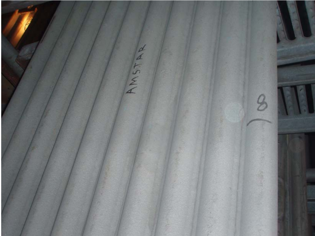
Figure 9. AmStar 888® cladding 39 ft Panel 3-4 installed in Pass 3 without passivator
