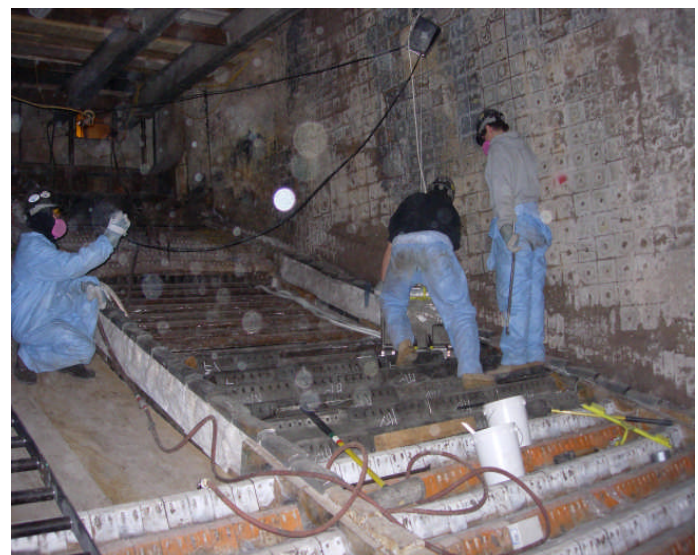
FIGURE 3 WINCH USED TO LOWER THE BLOCKS INTO PLACE
