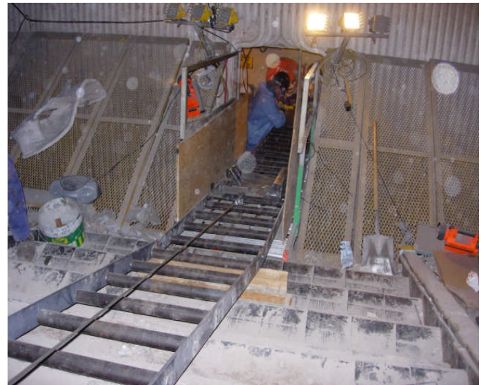
FIGURE 2 CONVEYOR USED TO TRANSPORT THE BLOCKS INTO THE BOILER
