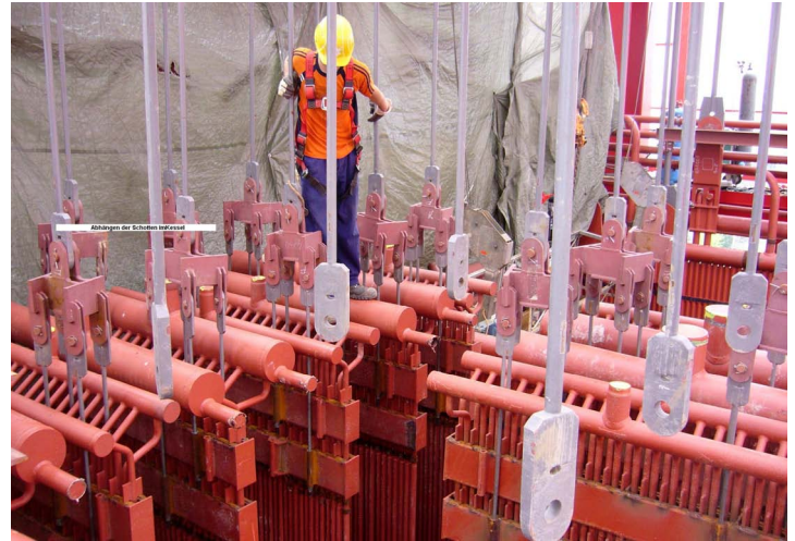
Figure 12 a – platen-type superheater
