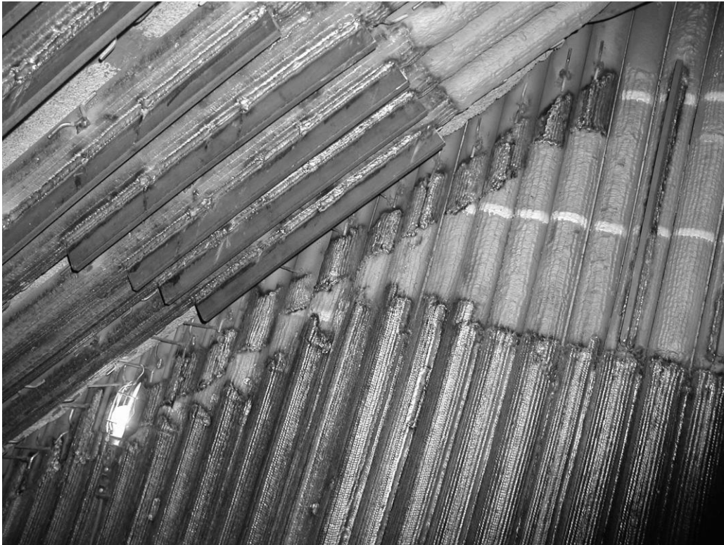
FIGURE 2- INSTALLATION OF SACRIFICIAL IRON BARS
