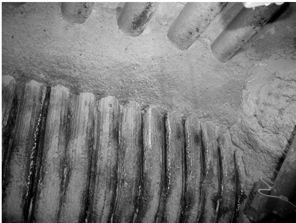
FIGURE 4- SURFACE TREATED WITH COPPER SULFATE
