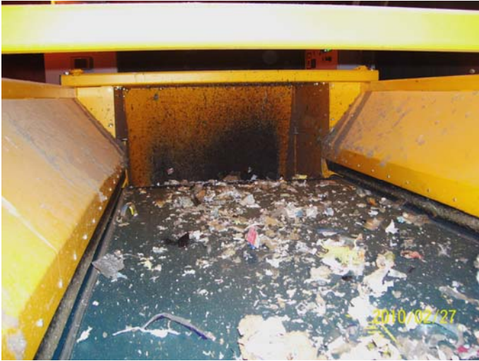
Figure 5. Process material on ECS conveyor
