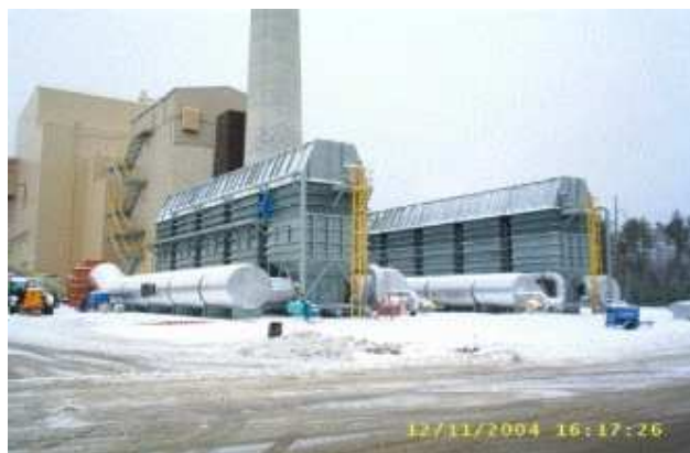
FIGURE 7: AN RSCR SYSTEM SHOWING TWO TRAINS OF 5 CANISTERS EACH
