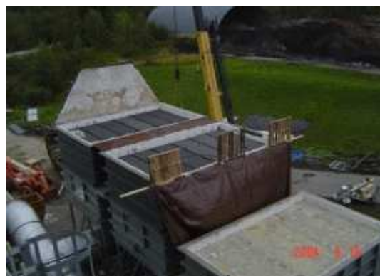
FIGURE 6: A THREE-CANISTER SYSTEM UNDER CONSTRUCTION
