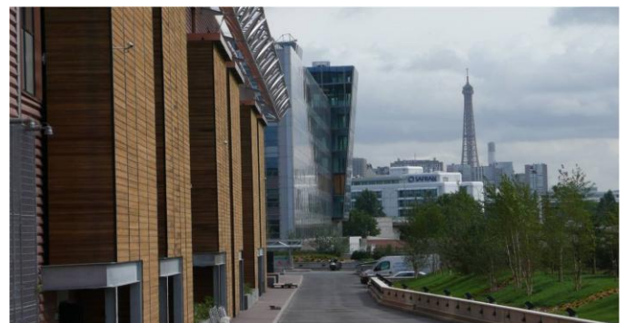
Figure 2, Rear of the plant looking at the Eiffel Tower 1
