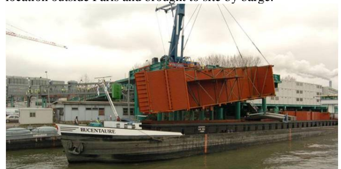
Figure 5, large components delivered to site
