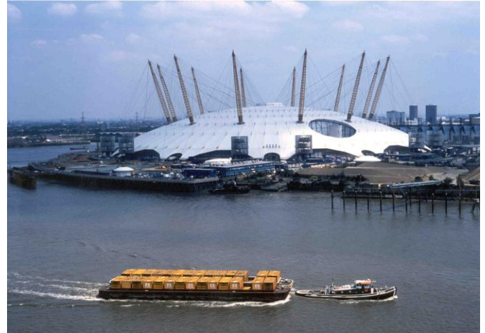
Figure 11, Waste transportation by barge on the Thames River
