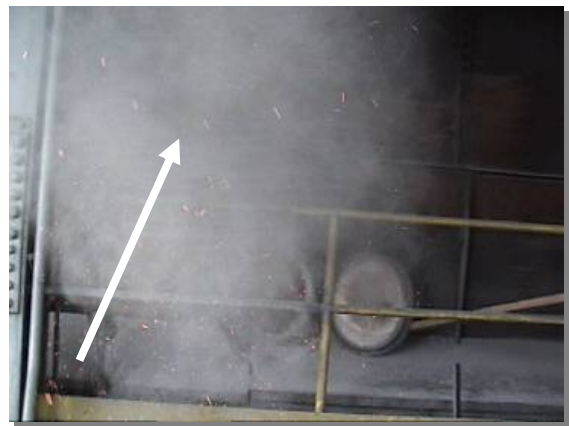
Figure 7: Ash Particles During Pressure Pulse Cleaning – Non-Line of Site Cleaning
