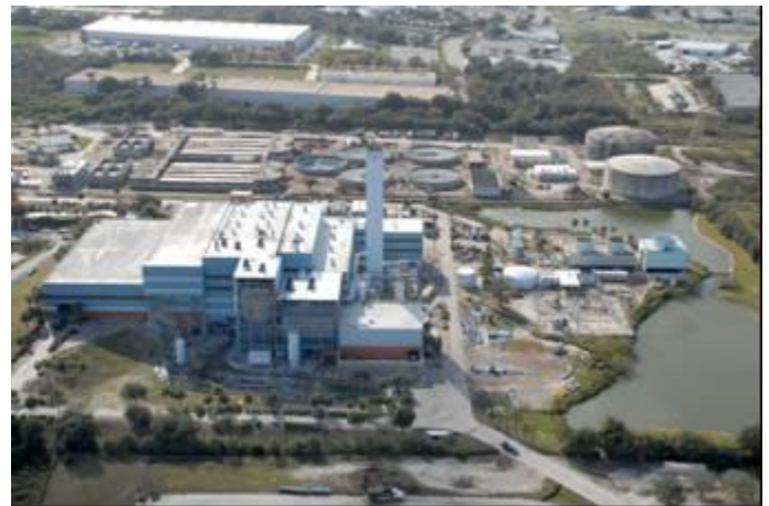
FIGURE 2 HILLSBOROUGH COUNTY EFW FACILITY EXPANDED CAPACITY 1800 TPD EXPANSION STATUS 1-9-09 COMPLETION SCHEDULED FOR 3RD QUARTER 2009. (PICTURE COURTESY OF COVANTA ENERGY)
