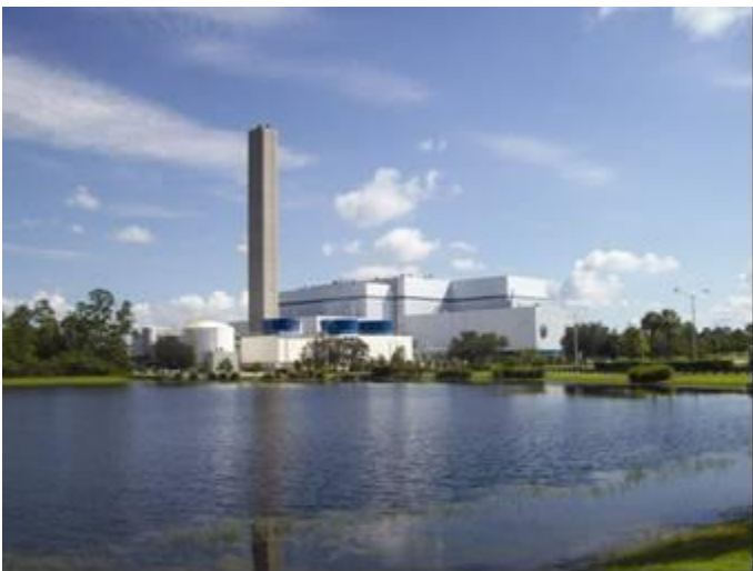
FIGURE 1 LEE COUNTY EFW FACILITY EXPANDED CAPACITY 1836 TPD EXPANSION COMPLETED OCTOBER 2007. (PICTURE COURTESY OF LEE COUNTY GOVERNMENT)
