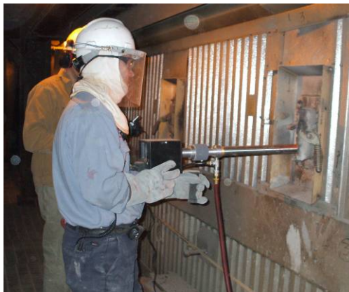
Mobile Infra Red Camera Inspection Unit 2 Covanta Hempstead, NY
