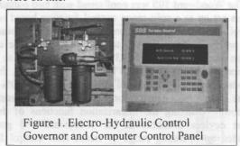
We then decided to investigate the capability of controlling a second valve from the Woodward 505 governor in a split-range configuration. The key question was whether the operation of a second valve, an automatic control valve working from the second digital controller on the 505, would
