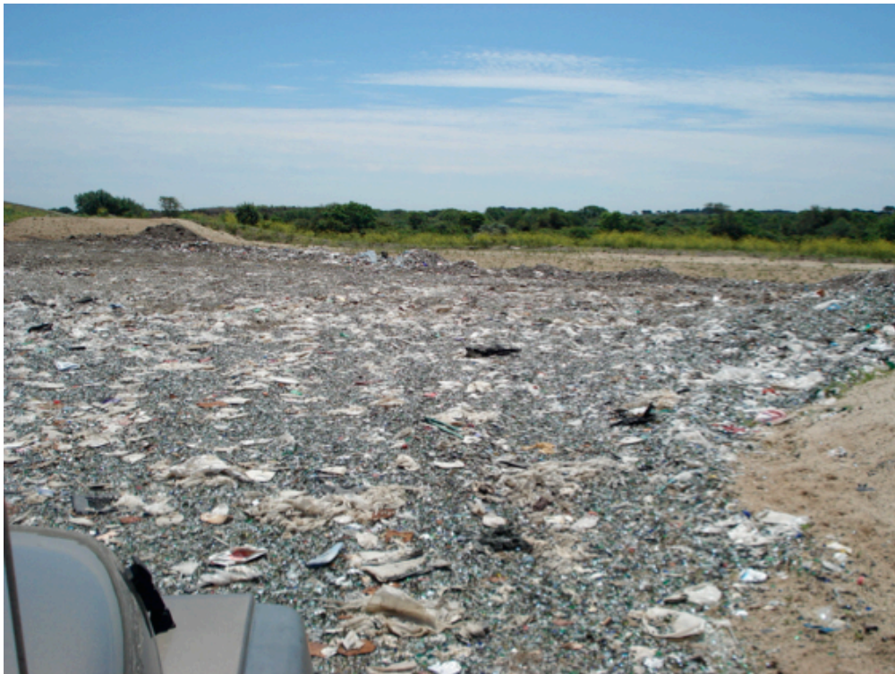
Figure 22: New landfill where glass is used as Alternative Daily Cover.
