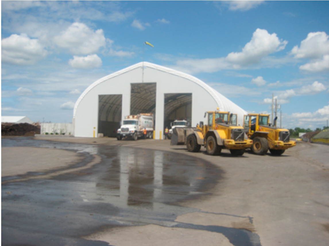
Figure 12: Tipping area with biofilter on the left (enclosed within walls). The organic waste is delivered here and the building is kept at a lower air pressure than outside, to prevent odors from being emitted.
