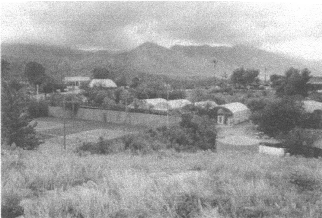
Tennis courts site looking southeast from hotel, visitor center is in the background on the right.
