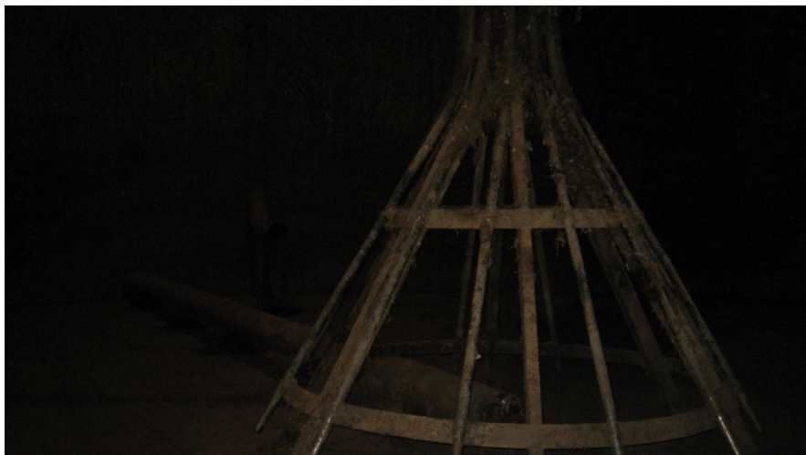
Figure 31 Inside of the one of the AD reactors (pipes for reintroducing the biogas), (photo by L. Arsova)
