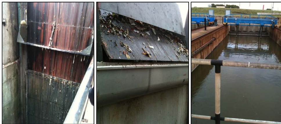
Figure 15, Wastewater treatment plant (WWTP) filters and ponds
