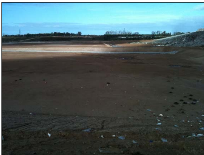
Figure 8, New cells (in construction)
