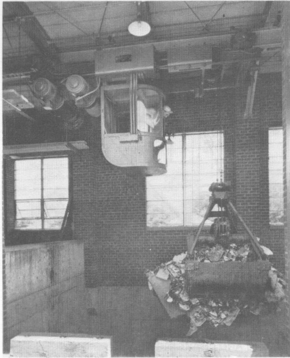
FIG. 5 MONORAIL CRANE WITH OPERATOR RIDING IN CAB WITH BUCKET FOR SMALL MUNICIPAL AND INDUSTRIAL INCINERATORS.
