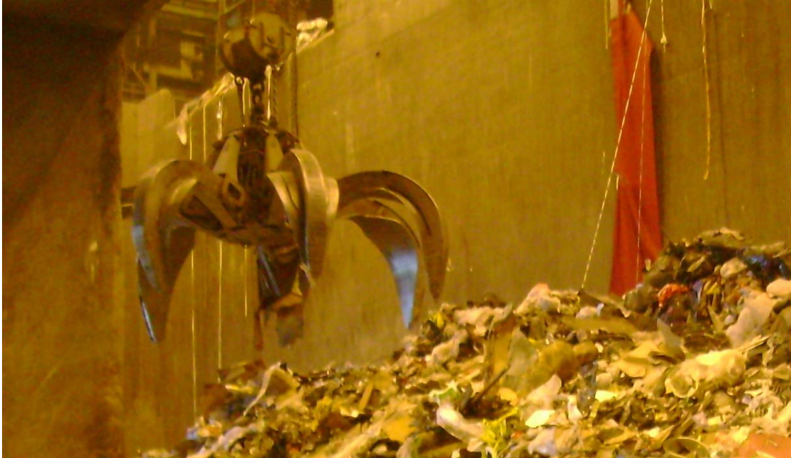
Figure 6: Claw prior to fluffing the pit
