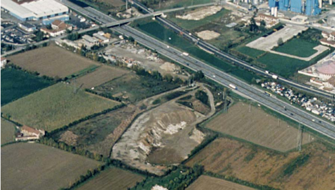
Figure 10: WTE Site before Construction
