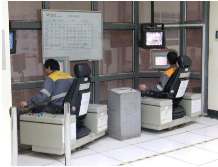
Picture 6 Likeng WTE plant operation room
