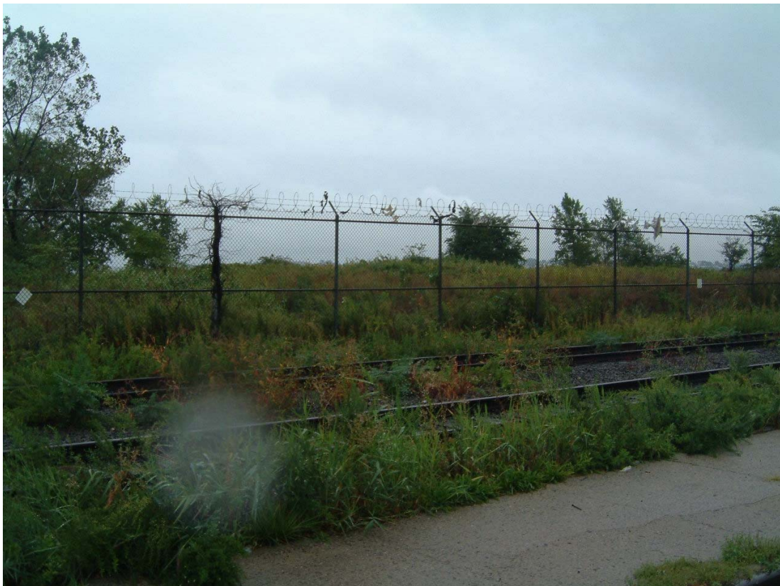
Figure 12. Front view of Hunt's Point property. Note rail access.
