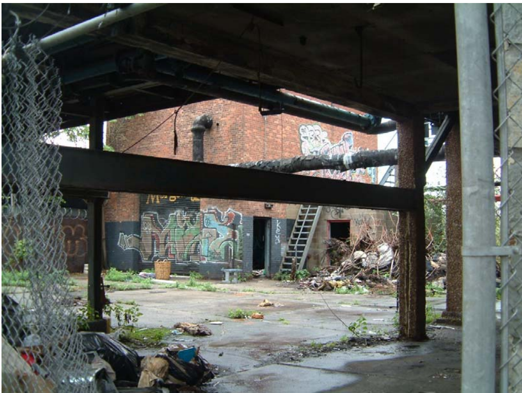
Figure 15. View of existing Brooklyn site.
