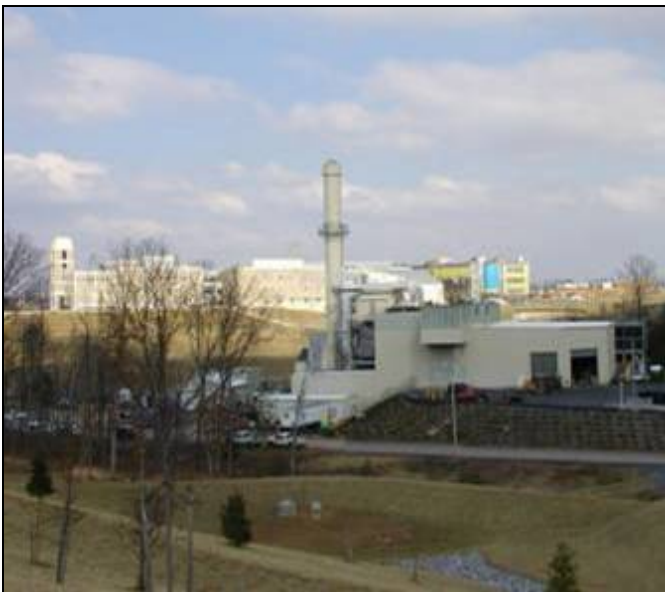
Figure 2.20 Harrisonburg WTE plant (114) .
