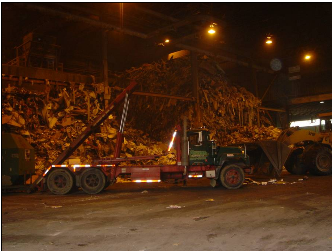
Figure 5.8 View of the tipping floor of Veolia ES (Montenay) Dutchess LLC WTE facility at Poughkeepsie, NY, USA (10) .
