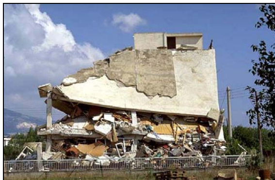
Figure 3.28 Photograph of demolished house at Nea Philadelphia (76) .
