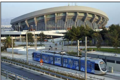
Figure 3.49 View of the tram (85) .
