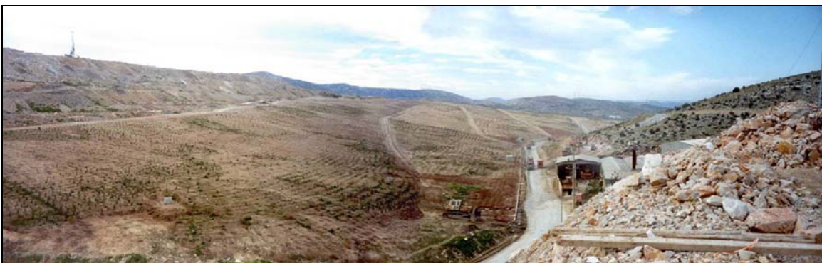
Figure 4.78 View of Ano Liossia site after restoration (136) .
