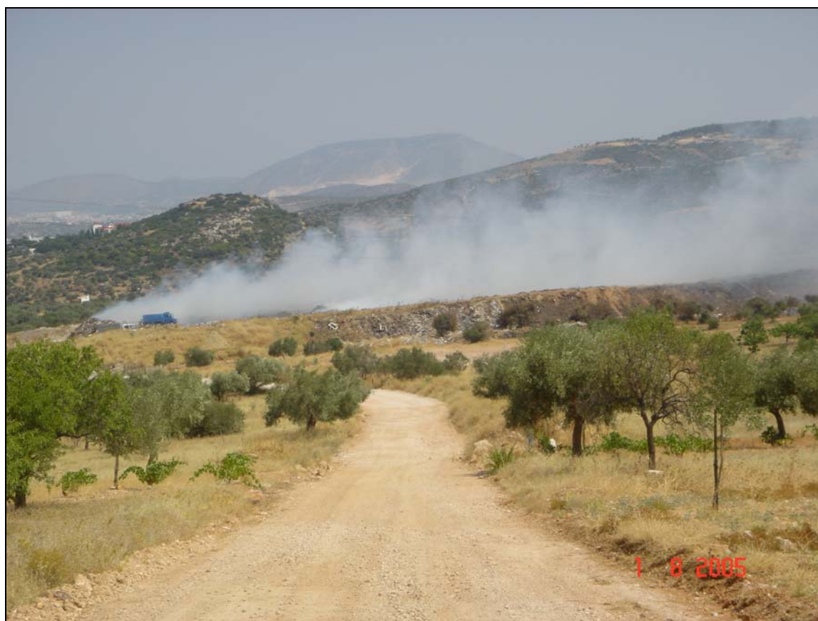
Figure 4.68 View of the eastern part of Cropia landfill.
