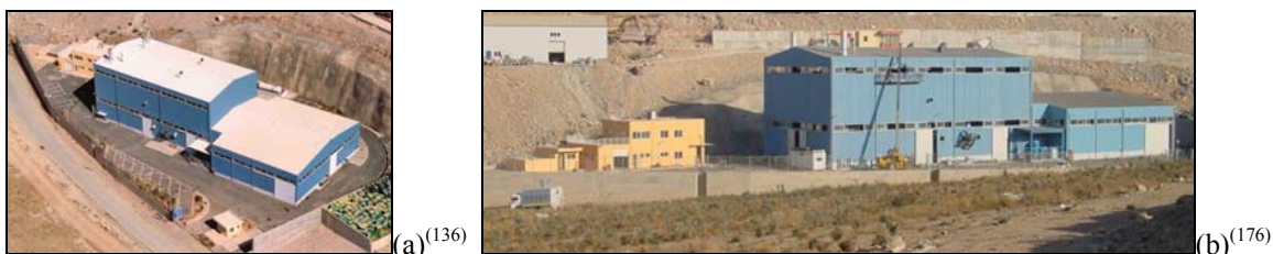
Figure 4.47 View of the MWI.
