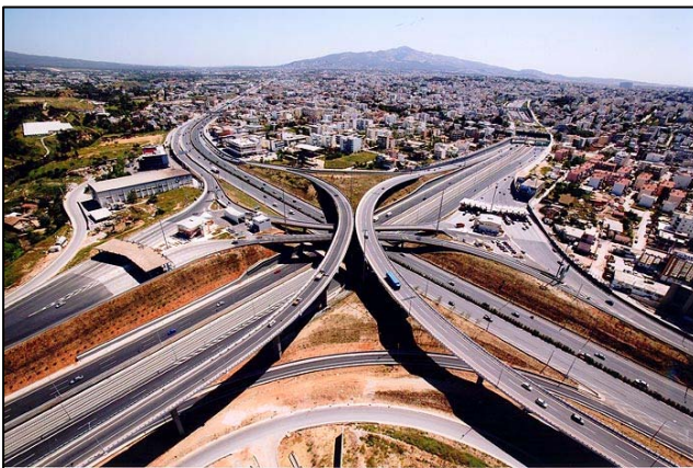
Figure 3.37 Photograph of Attiki Odos – PATHE Interchange (109) .
