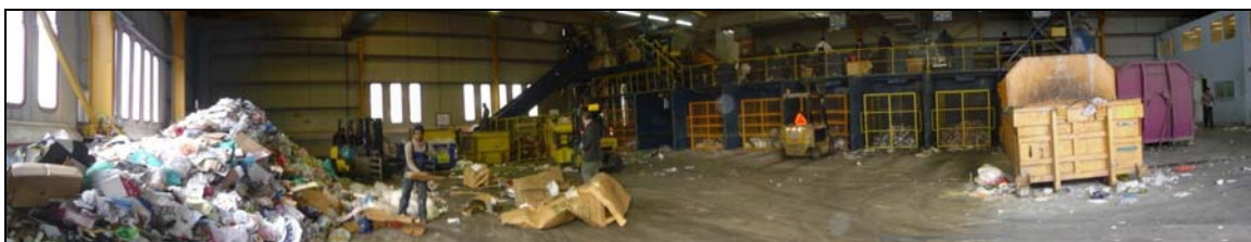
Figure 4.35 Interior of Maroussi HERRCo facility.
