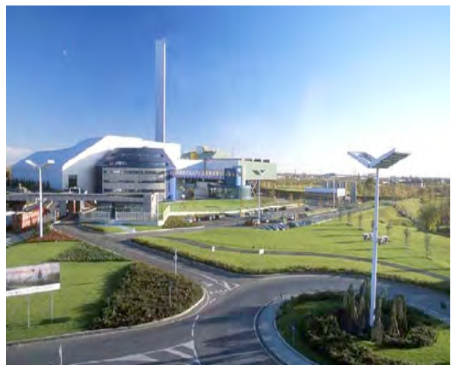
Figure 2: A waste-to-energy facility in Brescia, Italy {15}
