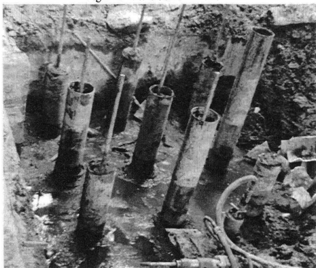
Figure 3: Mini-Pile Installation
