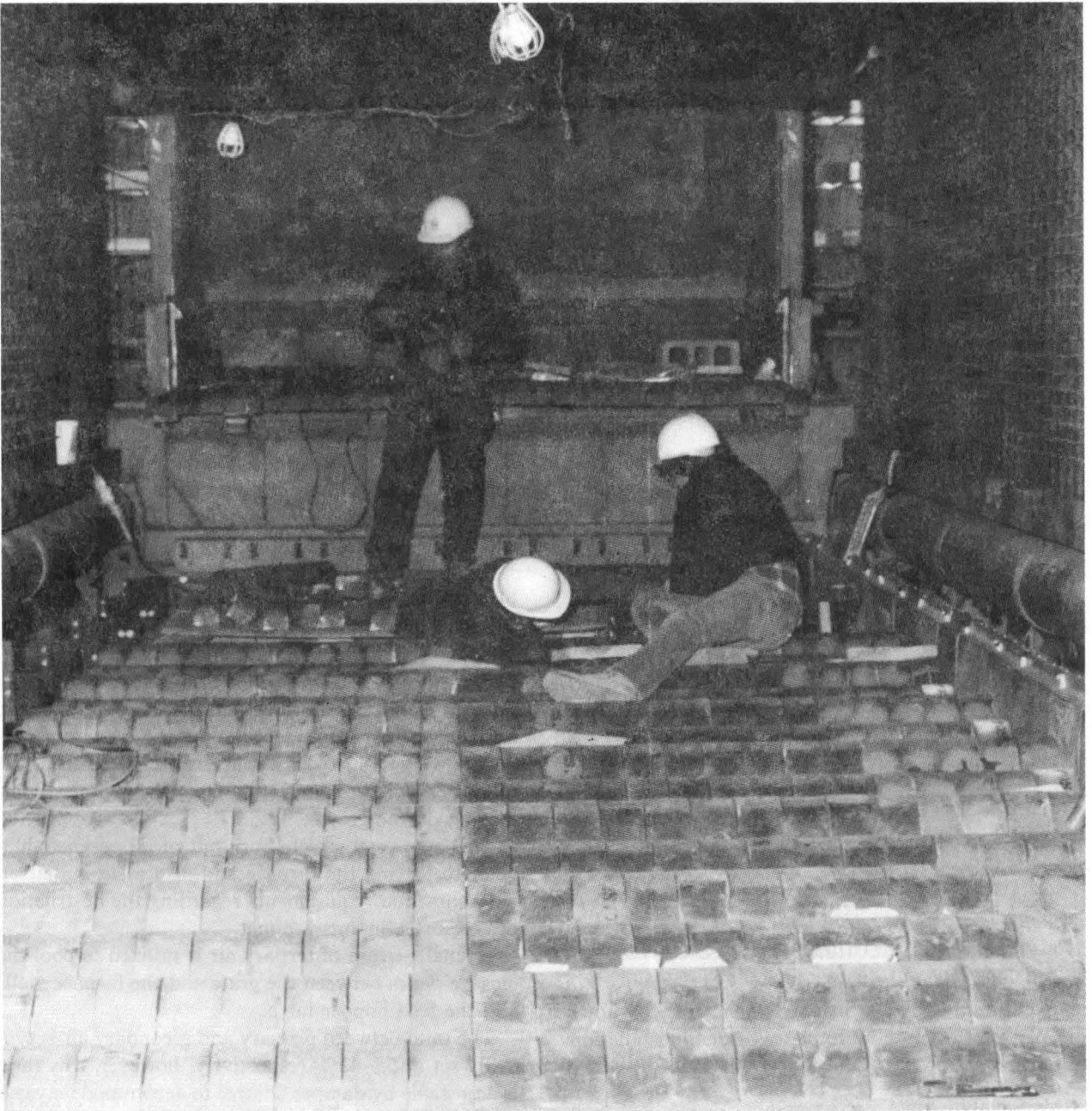
FIG. 7 WARREN COUNTY GRATE INSTALLATION
