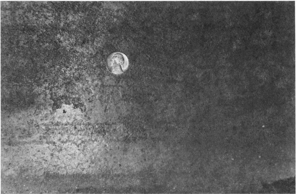
FIG. 11 CLOSE-UP OF CONVEYING SURFACE SHOWING PITTING CORROSION DEVELOPED AT DEPOSIT INTERFACE
