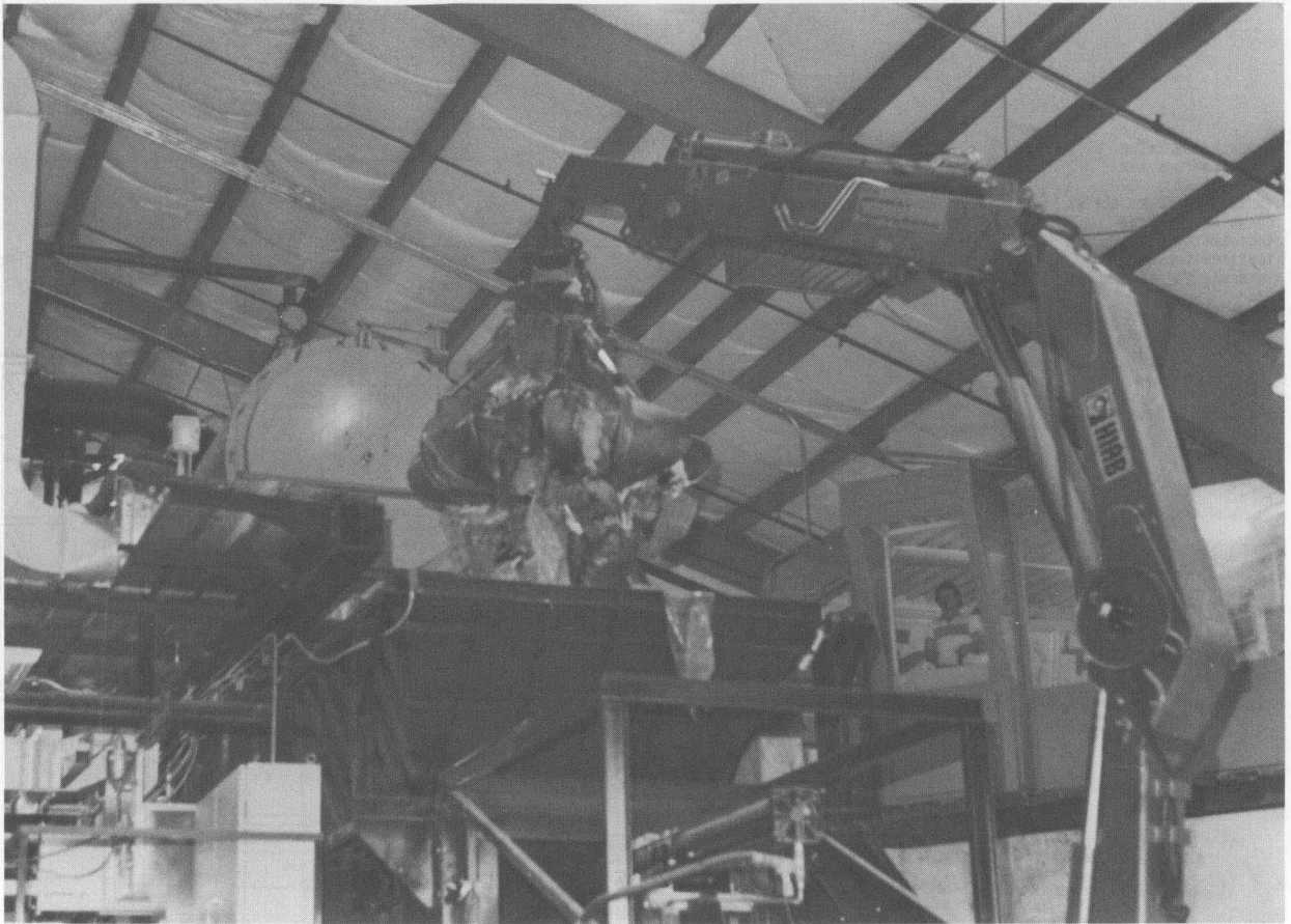
FIG. 5 VIEW OF KNUCKLEBOOM CRANE WHILE FEEDING INCINERATOR HOPPER
