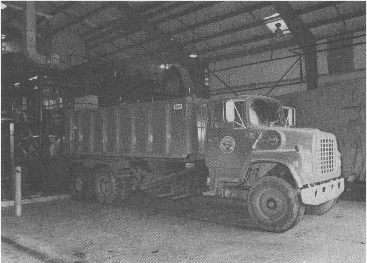
FIG. 9 VIEW OF SLUDGE DELIVERY TRUCK PREPARING TO DUMP SLUDGE INTO THE SLUDGE BIN IN THE HRI BUILDING
