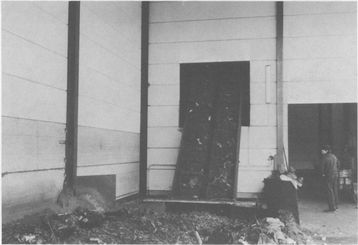
FIG. 5 DOSING BELT FEED CONVEYOR
