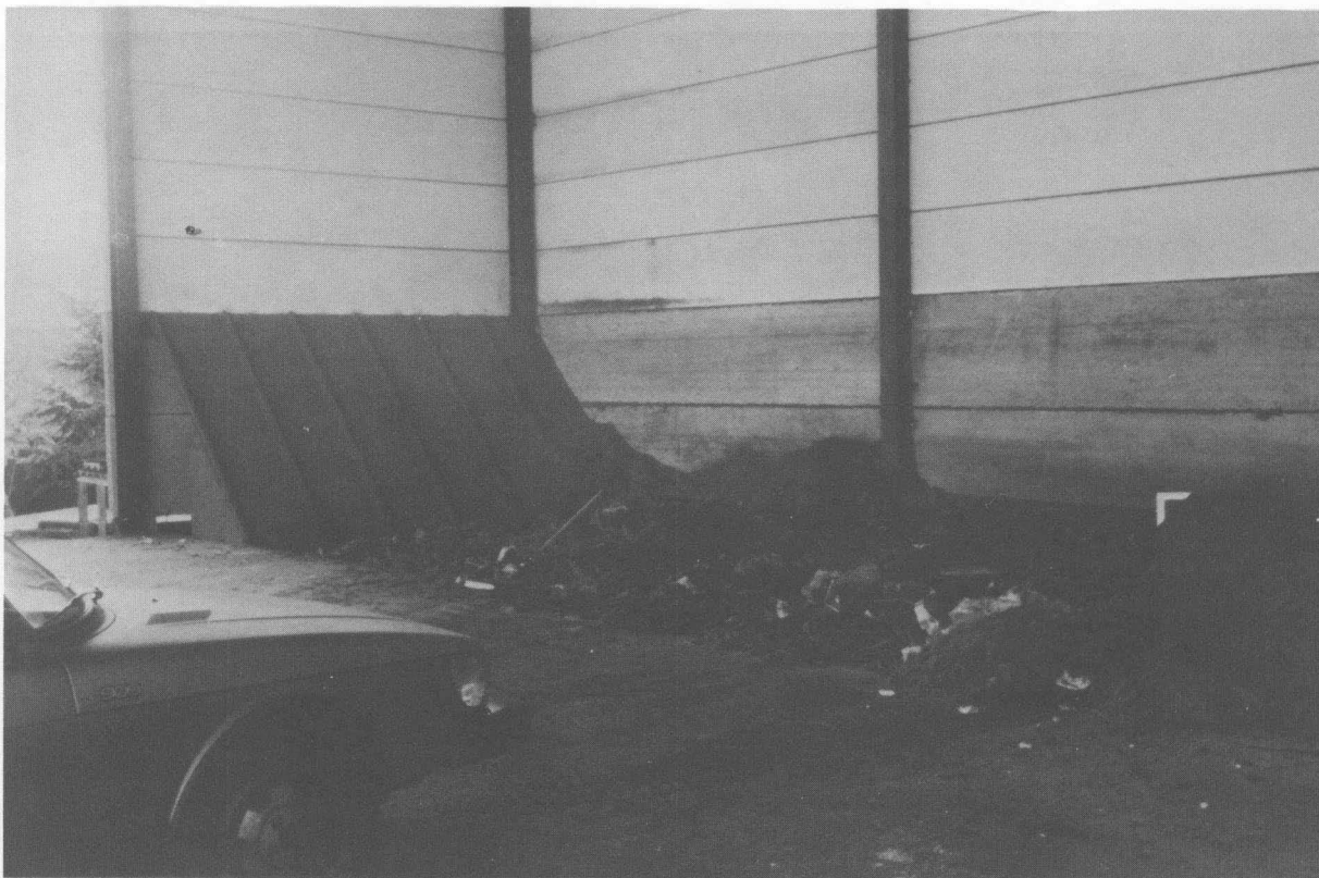
FIG. 4 LIVE BOTTOM STORAGE CONVEYOR
