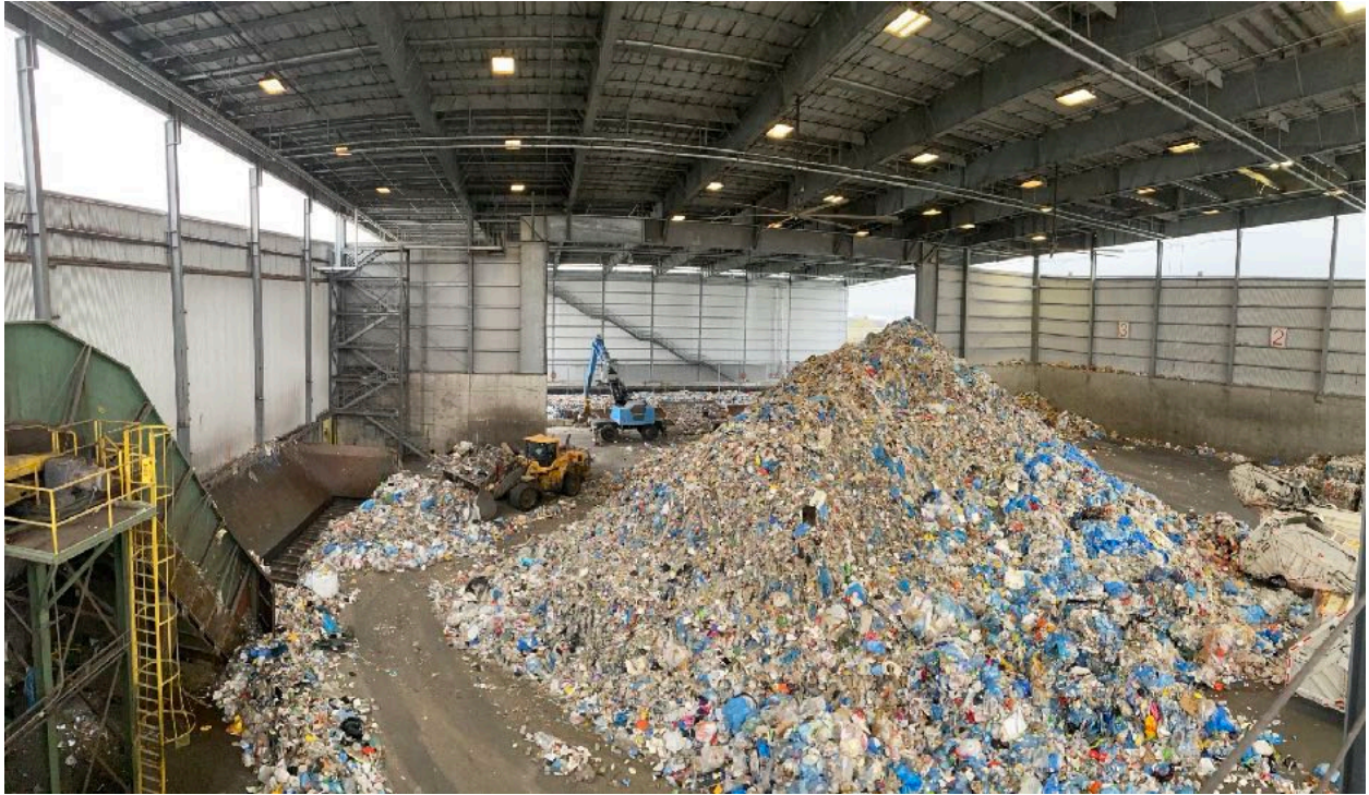
Tipping floor and the shredder to the left
