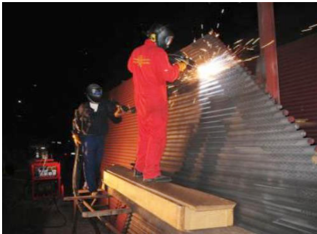
Refurbishing of SHT with Inconel 625 Arc Spray on site
