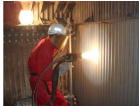
Refurbishing of SHT with Inconel 625 Arc Spray on site
